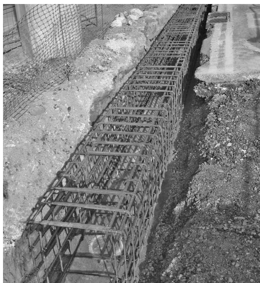
Figure 11.6. Torsionally reinforced continuous concrete beam foundation (showing reinforcing cage prior to placing of concrete)
