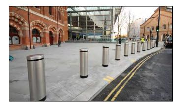
A VSB is usually positioned as far as possible from the vulnerable asset, typically near the existing or extended kerb line. If the barrier line is designed to be permeable to pedestrians the air gaps between structures should be no more than 1200mm. This is sufficient to allow wheelchair users and people pushing prams to permeate the barrier line.
